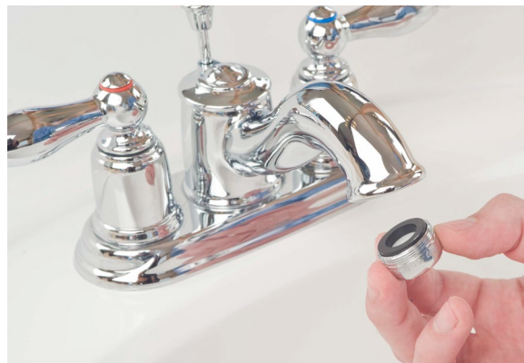
Removing an aerator for inspection
