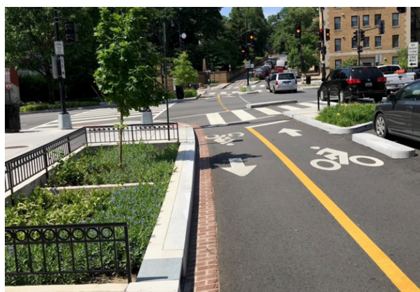
A "green street" uses practices such as porous pavement and bioretention to capture, infiltrate, and evapotranspire stormwater, preventing contaminated runoff from reaching local waterbodies.
