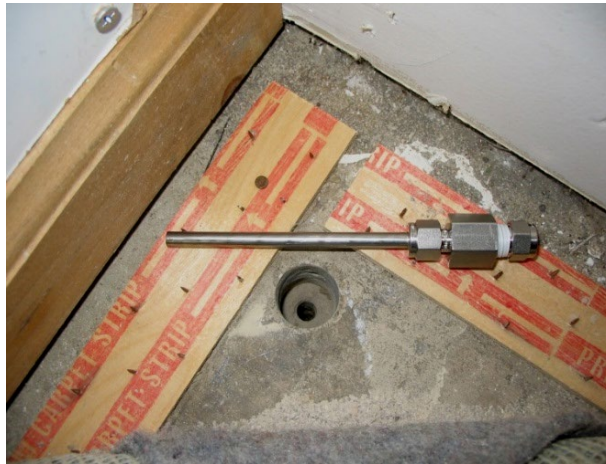
Figure 1: Assembled sub-slab port ready for installation
