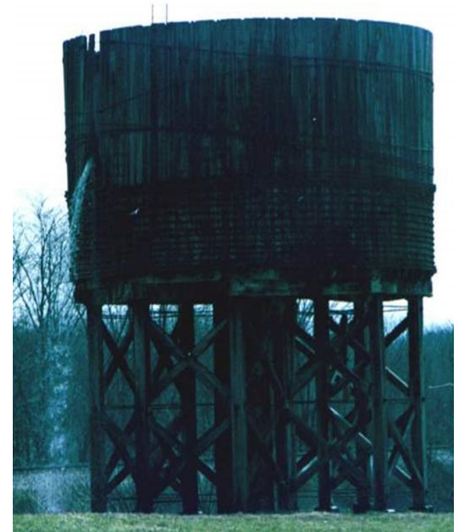
Ruptured Wooden Water Tower, March 1999
