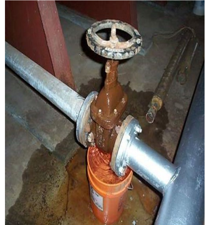
Leaking valve
