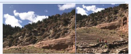
USEPA constructed erosion controls at the Mesa II mine to prevent mine waste from entering the Cove watershed. Before erosion control (left), and after erosion control (right).
