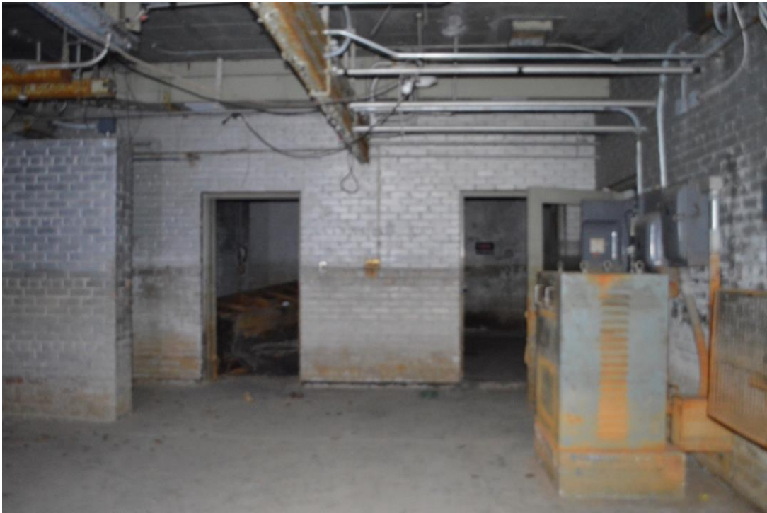
Photo 7 Looking south in basement where remediation is proposed, January 2023
