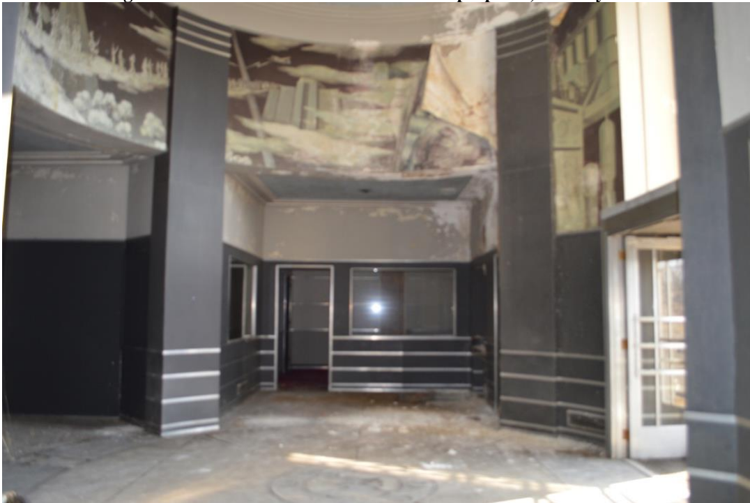
Photo 8 Looking east in main lobby, January 2023
