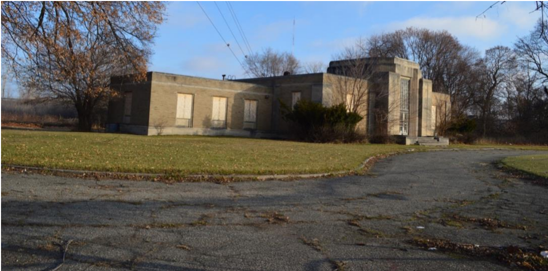
Photo 1 Looking northeast at WWJ building proposed for remediation and renovation, January 2023
