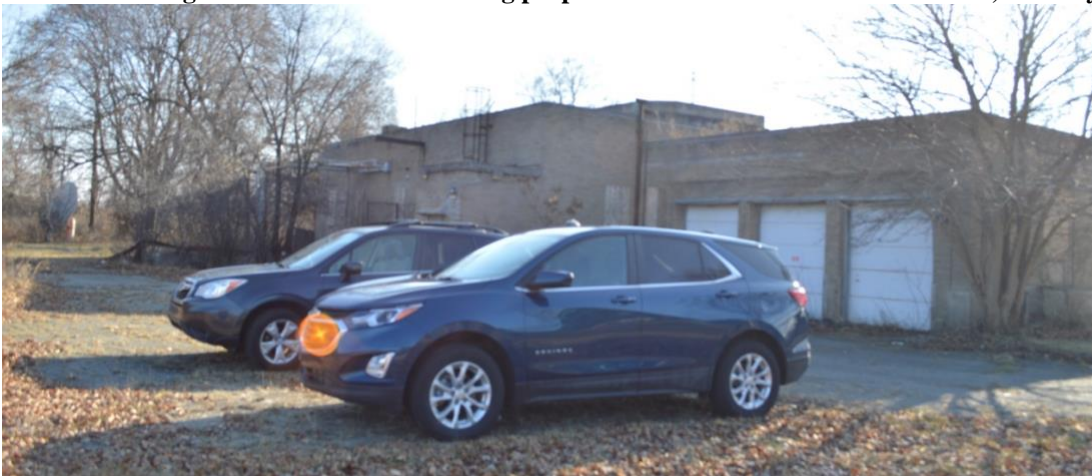
Photo 2 Looking southeast at rear of building at location of proposed addition, January 2023
