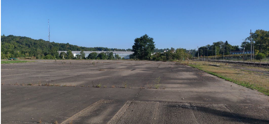
Photo No. 1 (091305): View looking north at transshipment pad located in Area 1. Green Street is beyond the railroad tracks on the right. Note tree growth within the capped area north of the pad.
