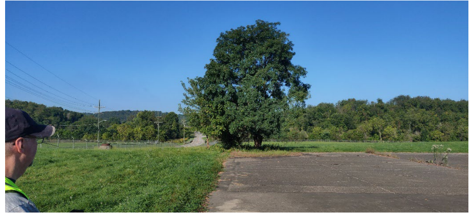
Photo No. 2 (091313): View looking west at transshipment pad located in Area 1. Caldwell Ave. is to the left of the property fence. Note tree growth within the capped area west of the pad.
