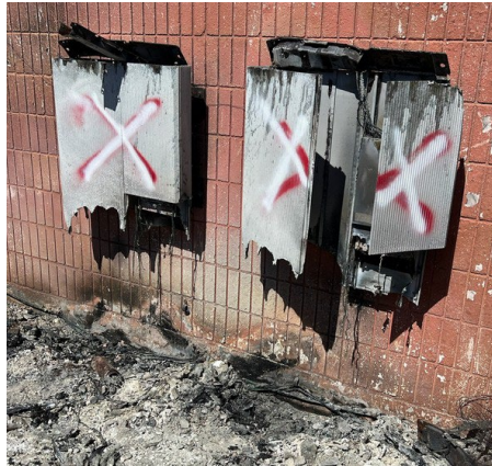
Puting slash na tumatakip sa pulang pintura = Na-clear na lithium battery power walls o photovoltaic equipment.
