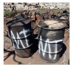
White "MT" mark = Fuel tank contents were transferred, and tank left in place.
