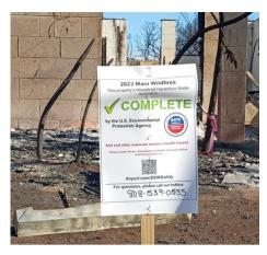
White signage and stake = a site has been cleared of hazardous material (HM) and is completed.
