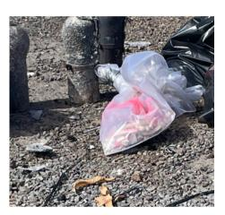
Pink paint = Suspected asbestos containing material.
