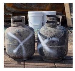
White paint or "X" mark = Empty HM containers or containers to be left in place and removed in Phase 2.
