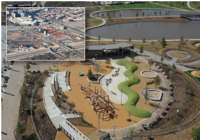
Scissortail Park in Oklahoma City before (inset) and after Section 128(a) funded cleanup oversight and redevelopment. Credit: scissortailpark.org .
