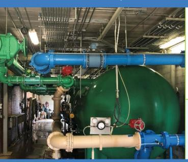
After testing revealed manganese levels to be three times higher than EPA's public health advisory level, the City of West Point used **\$3.5 million in DWSRF funding** to replace water treatment plant filters and upgrade system controls. They also installed variable frequency drives to better control water flow. Following the water treatment plant improvements, manganese levels were brought below the secondary maximum contaminant level (MCL).
