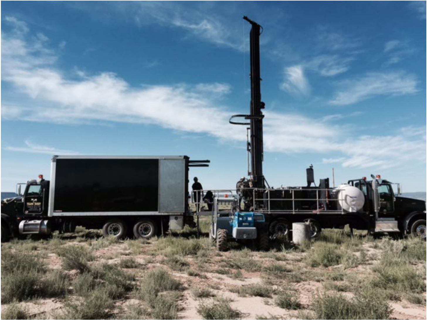
Drilling rig being used to install sampling wells.
