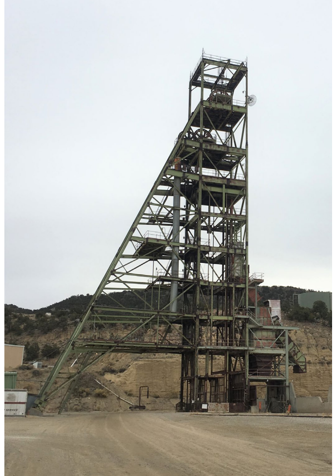
Head frame at Mt. Taylor before demolition
