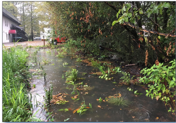
Figure 2. A rain garden installed on CCTHITA property captures and treats stormwater runoff.
