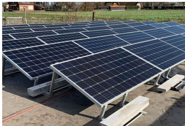
Example of a ballasted racking system for solar. Photo courtesy of NREL.
