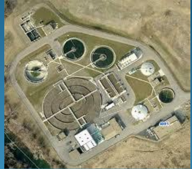
POTW is more than just the treatment plant
