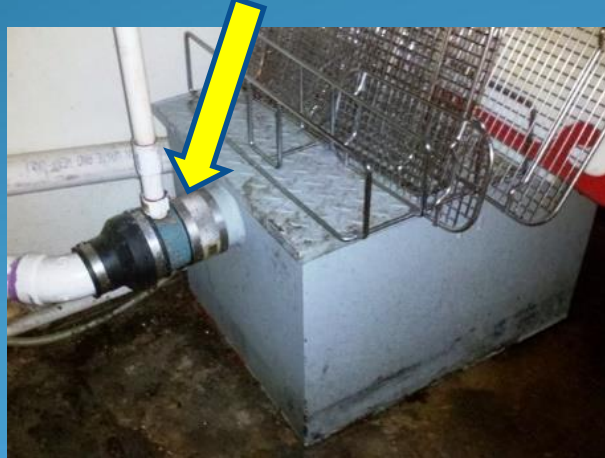
External Flow Restrictor & Vent Pipe
