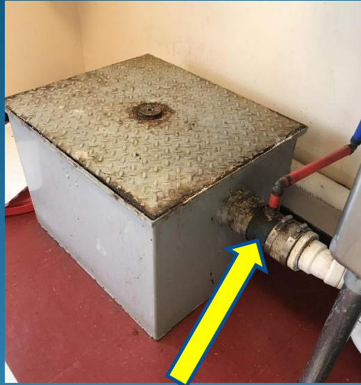
External Flow Restrictor & Vent Pipe
