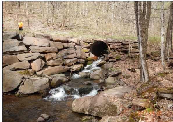
Figure 2. Looking upstream at the old deteriorating metal culvert outlet pipe and constructed outfall protection.
