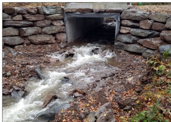
Figure 3. Looking upstream at the newly installed box culvert outlet and the stream grade control structure.
