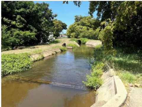
Photograph 1: View of the irrigation channel after the intake location.
