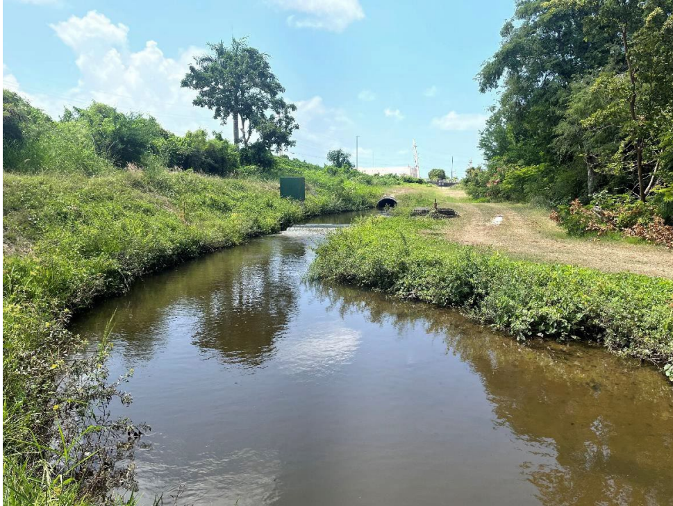
Photograph 6: View of the irrigation channel that conveys raw water from Patillas Lake, which is a reservoir.
