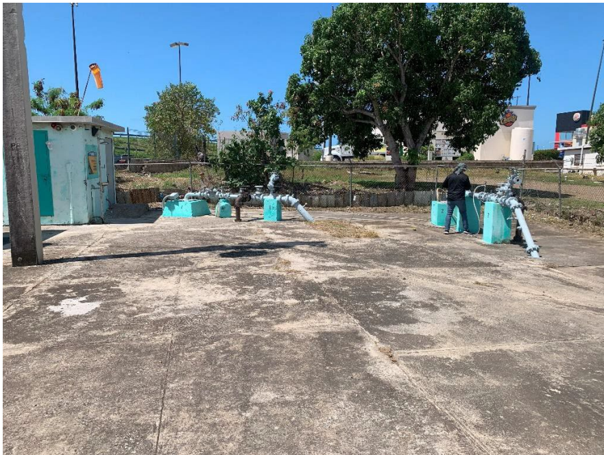
Photograph 8: View of PRASA personnel working at the Godreau 1 and 2 Wells.
