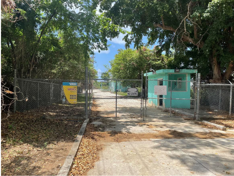
Photograph 5: View of the Rexmanor Pump Station entrance located at latitude 17.98132°, longitude -66.10133°. The Pump Station transports raw water from the intake location to the Guayama DWTP.
