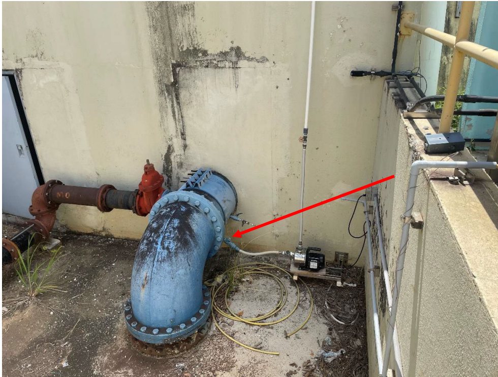
Photograph 3: View of the location from where the effluent sampling faucet receives treated water. Effluent samples came from the outlet of the storage tank and the beginning of the distribution line located at latitude 17.99053°, longitude -66.11182°.
