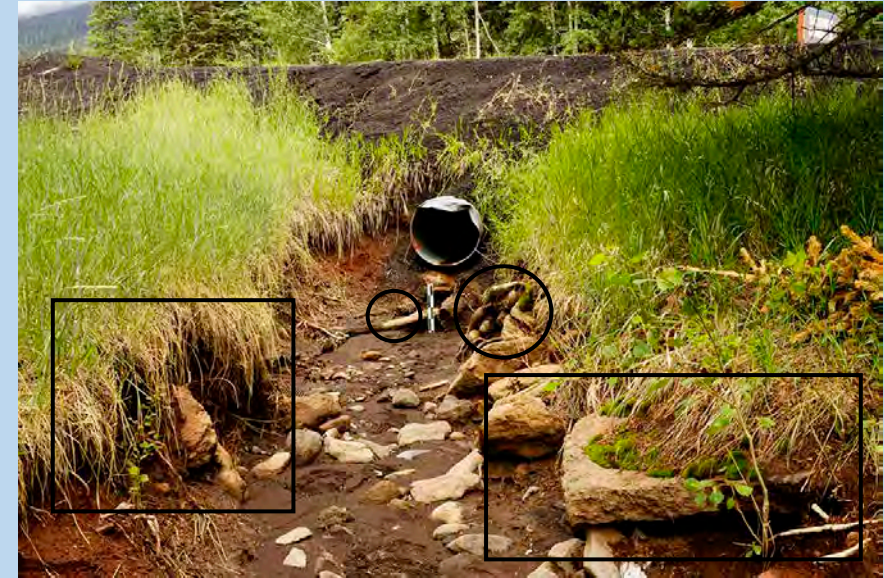
Upstream views of lower drainage system at and downstream of culvert. Upper left 9/20/2020 upper right 7/27/2021, scale 50 cm long with 10 cm (~4 inches) divisions. Common features are circled. Gully is deeper and substantially wider (rectangles).
