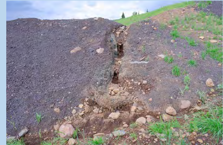
Left, rills were eroded into south and west-facing sides of parking lot during late July runoff. Right, rill of farthest west of two channels.
