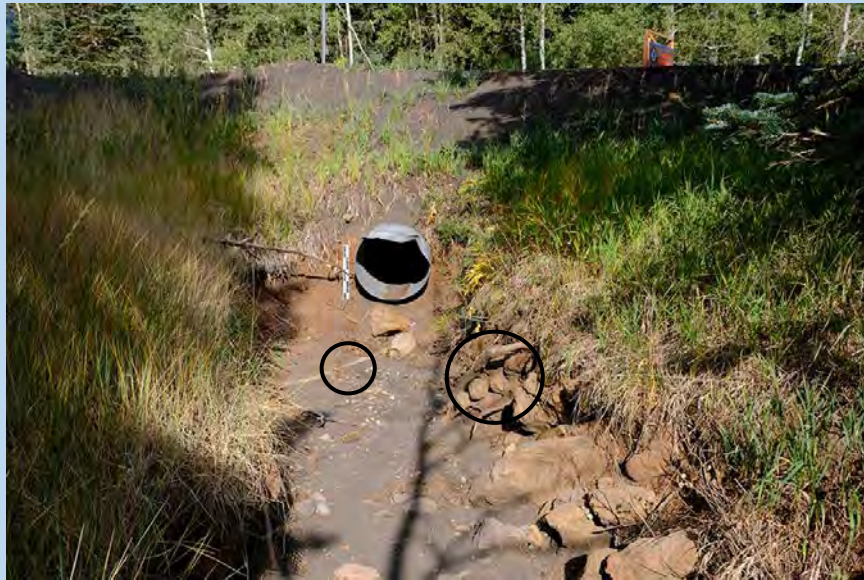
Upstream views of lower drainage system at and downstream of culvert. Upper left 9/20/2020 upper right 7/27/2021, scale 50 cm long with 10 cm (~4 inches) divisions. Common features are circled. Gully is deeper and substantially wider (rectangles).
