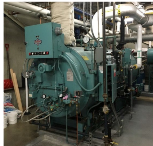
Commercial boiler that uses energy to generate steam for building heating
