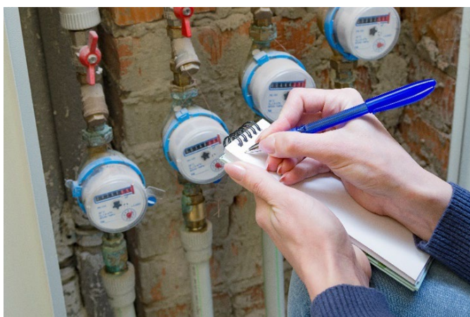
Reading facility submeters
