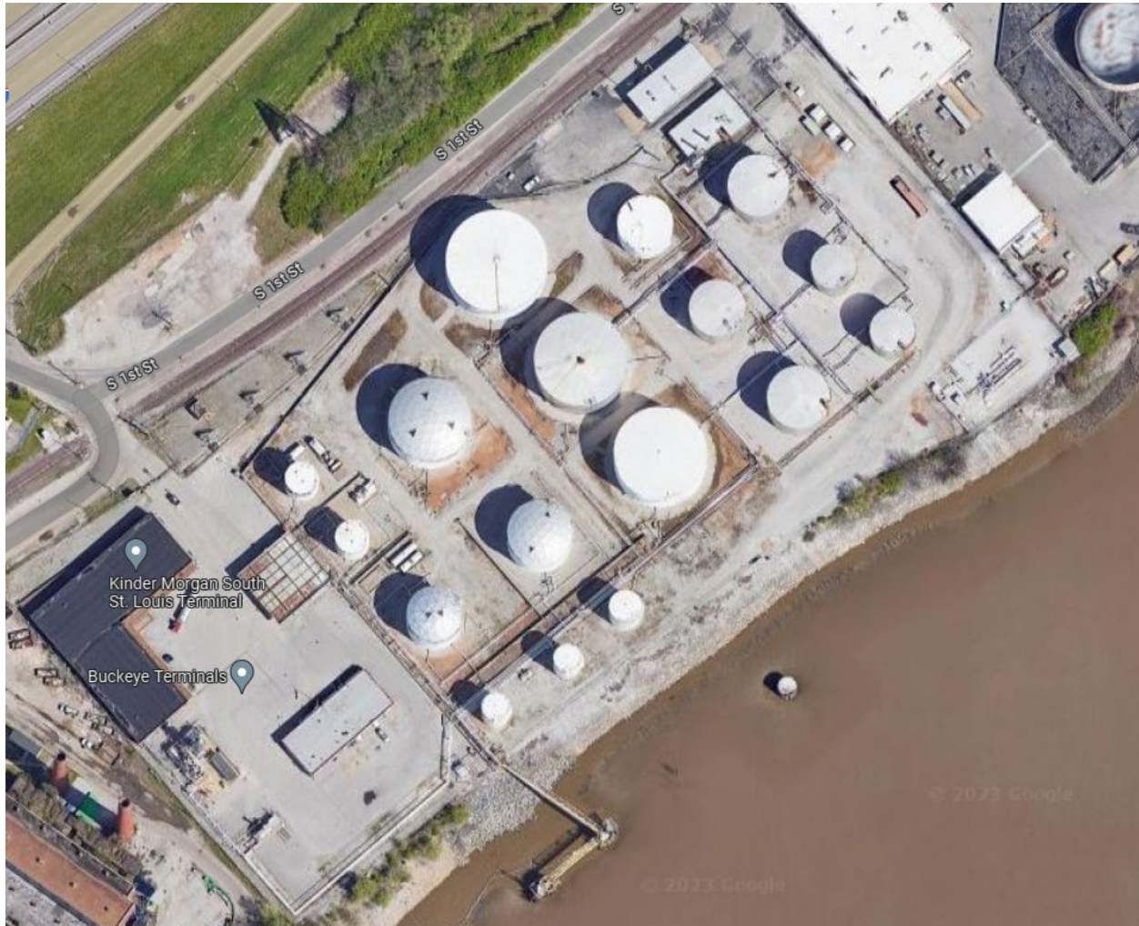
Figure 1: Satellite image of the Buckeye Terminals – South St. Louis facility in St. Louis, MO.
