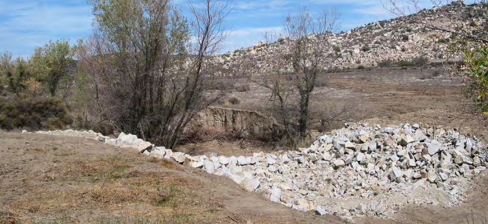
Diabold Creek detention structures that follow traditional Kumeyaay practices on the Campo Indian Reservation in San Diego County in 2002. Photo credit: Paul Ganster
