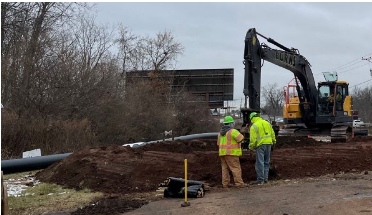
Fig. 6 Water transmission main was installed in the Berlin Water Control Commission small water system to replace aging infrastructure. The project was funded by the DWSRF.
