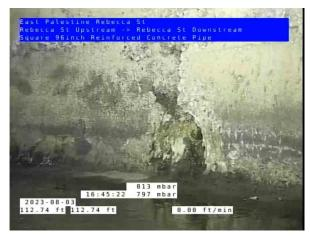
Rebecca St Upstream-Rebecca St Downstream\_00b267ff-80a7-4010-8d32-b657c569c33a\_202308 06\_172205\_377.jpg, 00:06:46, 112.73ft Fracture Multiple from 1 o'clock to 5 o'clock, Start
