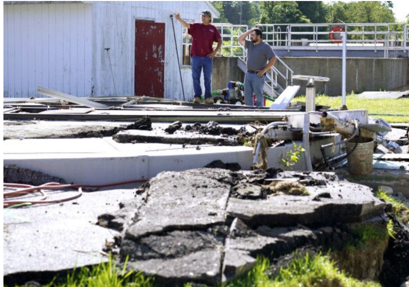
Figure 2: Ludlow Wastewater Treatment Plant (photo August 2, 2023, taken after July storm event) 16
