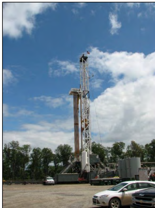
Figure 25. Well Pad development is ongoing in the region: Credit DCNR.
