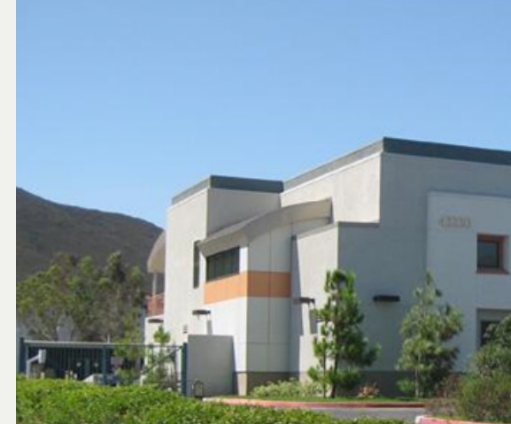
A. FACILITY POWER
