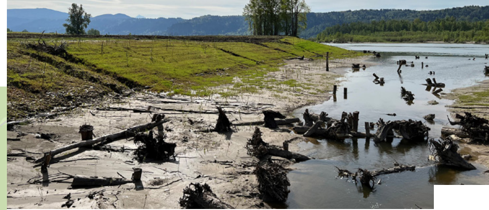
A restoration project removed over two miles of a levee and an elevated canal to reconnect Gibbons Creek to its floodplain and the Columbia River in WA.
