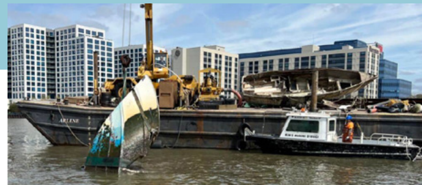
Debris is removed by crane in the New York-New Jersey Harbor.
