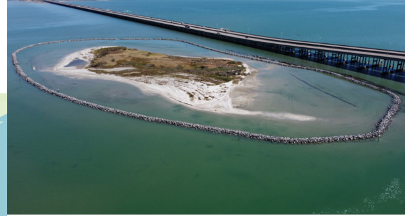
An island in Nueces Bay in Texas. A rock breakwater protects the island from erosion and provides nesting habitat for coastal waterbirds
