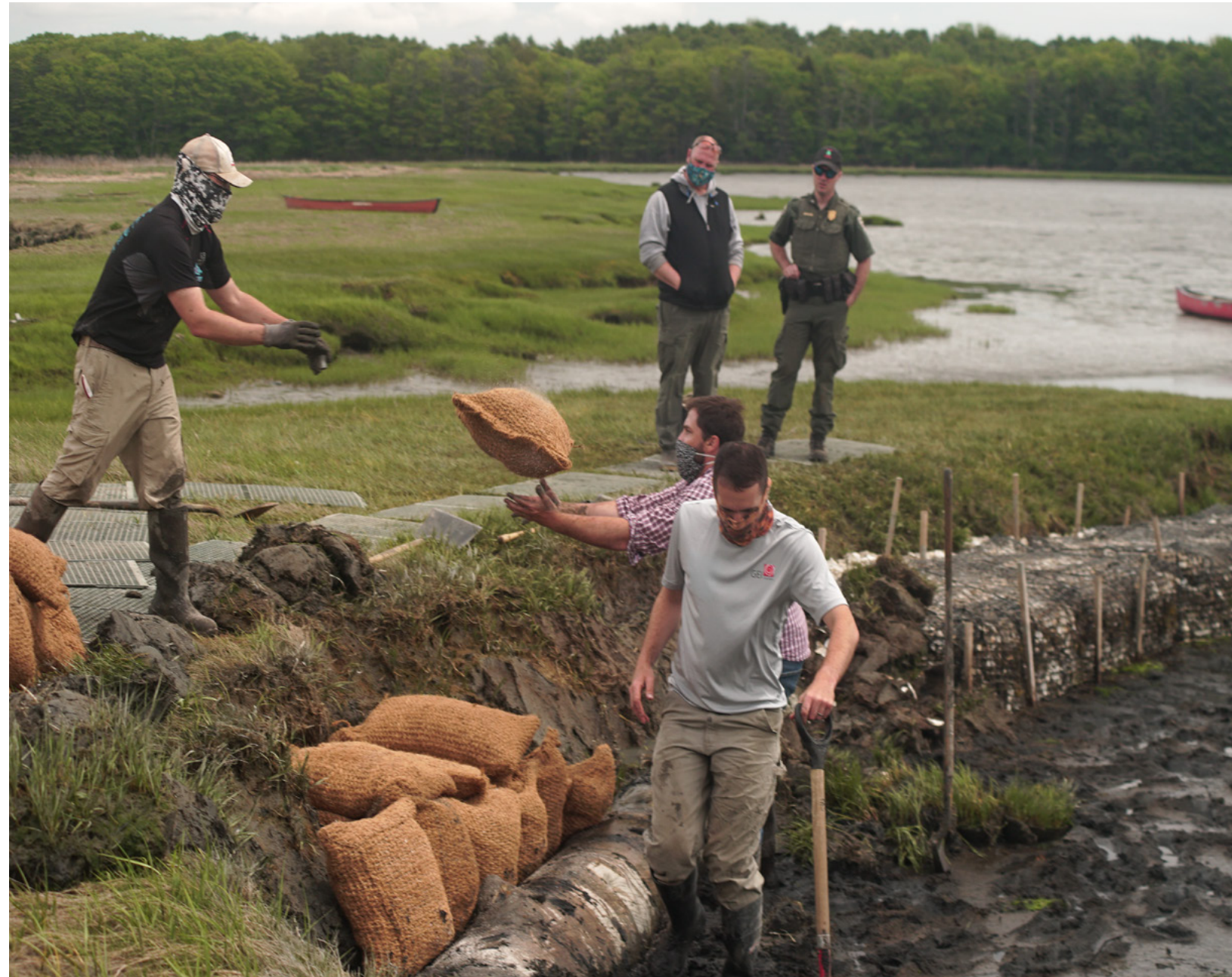
Volunteers constructing a Living Shorelines demonstration site in Brunswick, Maine.
