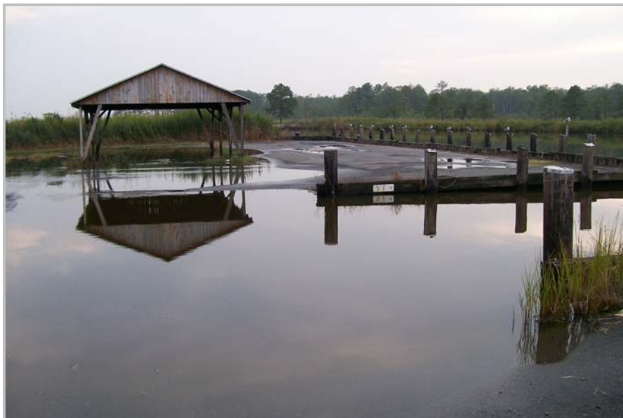
Boat ramp, pavilion, and parking lot inundated by spring high tide. Transquaking River at Bestpitch Ferry Road. October 27, 2007
