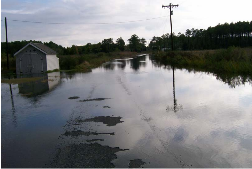
Aisquith Island Road during a spring high tide and strong south winds. The tide of Charles Creek was one foot above mean high water elevation. Crapo, Maryland October 27, 2007
