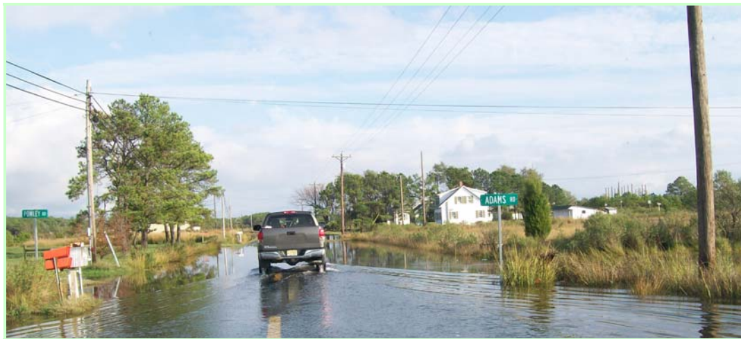
Wingate Bishops Head Road at its intersection with Adams and Powley Roads. High tide on Hearn's Creek has flooded all three roads. Wingate, Maryland October 27, 2007
