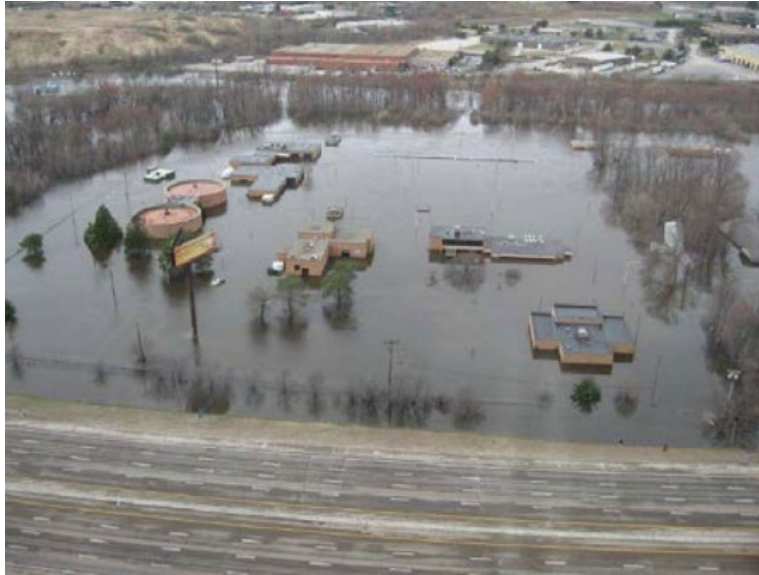
Figure 1: The flooded Warwick wastewater facility on Wednesday, March 31, 2010. (State of Rhode Island)
