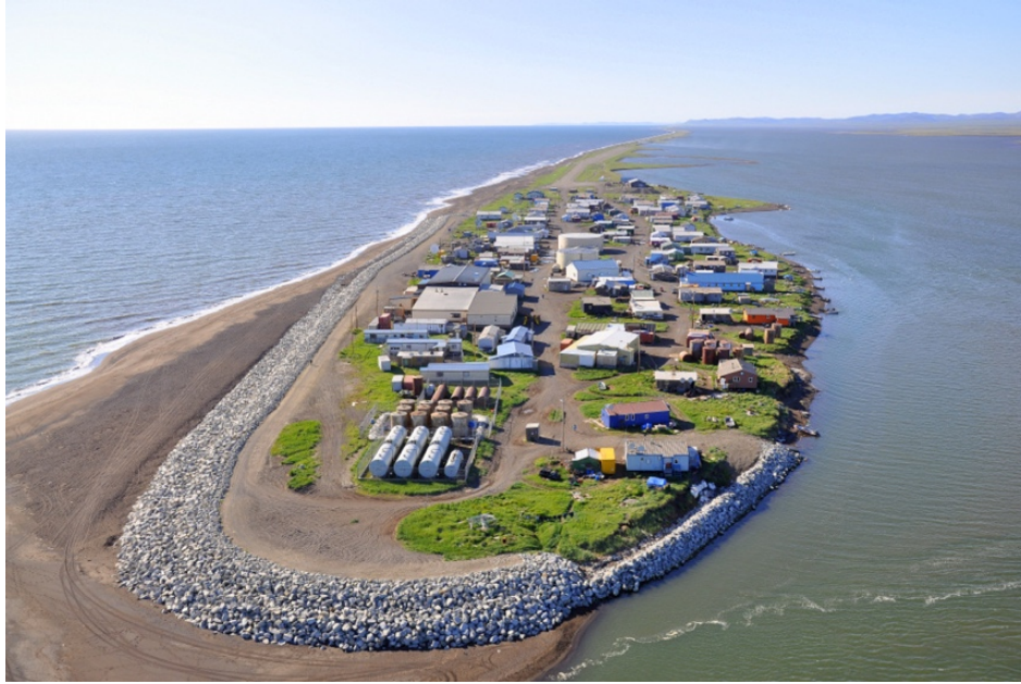
Kivalina's Rock Revetment 121
