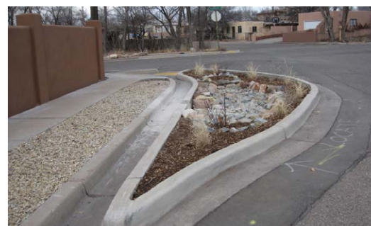
A small bioretention system at the intersection of Espinacitas and Hopewell streets in Santa Fe, constructed in 2016 through the retrofit of an existing vacant curb median. Photo: Santa Fe Watershed Association
