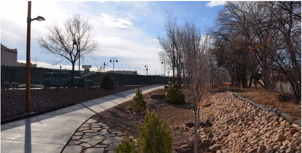
Figure 1. Acequia underpass bioretention. Source: City of Santa Fe
