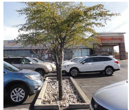
Curb inlets to tree trench pavilions in an Albuquerque parking lot. Photo: Tess Houle
