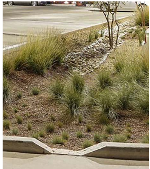
A bioswale with bioretention/bioinfiltration taking stormwater from a parking lot. Photo: Arid LID Coalition
