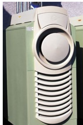
Figure 3-5. Microturbine
