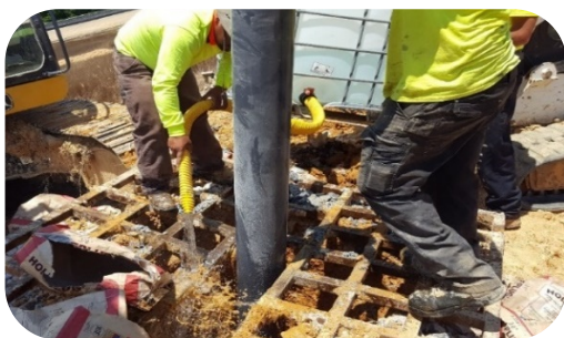
Hydrating bentonite to seal a well
