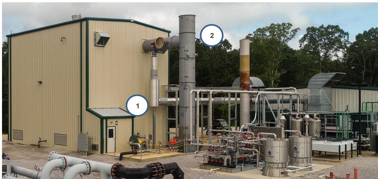
Figure 3-12. Concentrator Type of Leachate Evaporator – Heartland’s Low Momentum-High Turbulence (LM-HT®) Evaporator Using Heat from Both (1) Engine Exhaust and (2) LFG Flare
