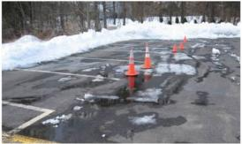
Accumulation of standing water in a parking lot after snow melt. Comparison between porous pavement (left) and regular pavement (right). Source: UNH Stormwater Center
