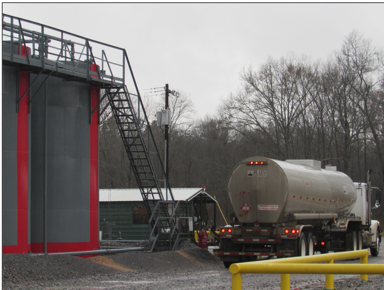
Figure 3-13. Truck Loading Operations
