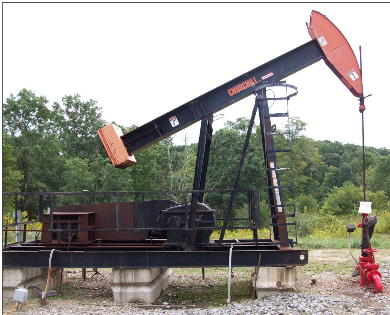
Figure 3-2. Coalbed Methane Dewatering Pump
