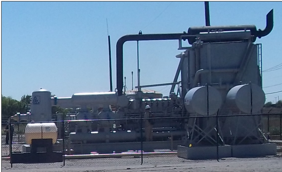
Figure 3-10. Lateral Compressor Engine
