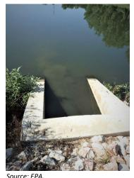
Image 1. Sludge accumulation at a transfer structure.
