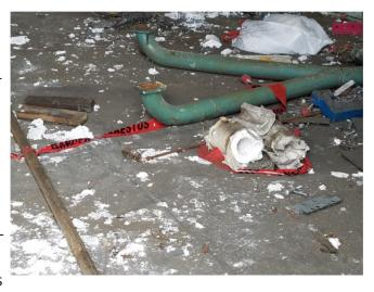
insulation (TSI). The survey noted that the asbestos-containing TSI was "friable" (that is, easily crumbled with hand pressure), and, therefore, "will require removal by a licensed asbestos contractor prior to any renovation or demolition activity that would directly impact these materials." Mischenko was provided a copy of the survey report on or about December 4, 2017.
