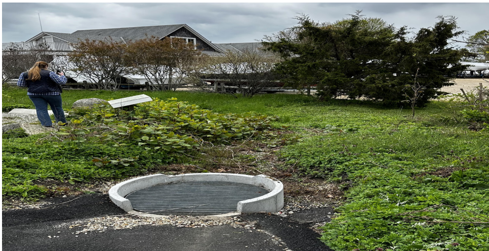
Newly installed rain garden turret to improve functionality of existing bioswale. The large stones in the foreground of this image demonstrate the high volume of stormwater in this area and the importance of functioning stormwater controls. Photo credit: SNEP
