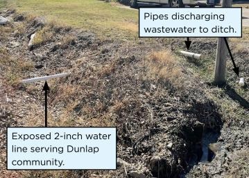
Figures 3 and 4. Exposed water lines in Dunlap.
