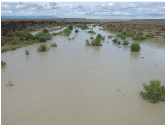
September 11, 2002 – View from Navajo Route N36 Bridge.
