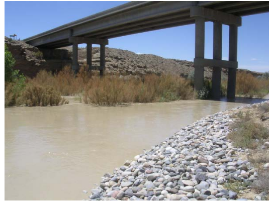
July 28, 2011 – At Navajo Route N36 Bridge.
