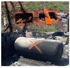
Orange paint = Septic system location, damaged transformer, or high hazard item stay left on site.
