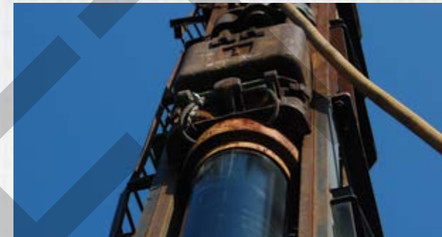
Vulcan 01 Impact Hammer Driving 16" Diameter SUPERPILE®
