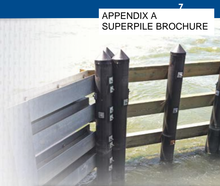
Margate Bridge Installation, Margate New Jersey
