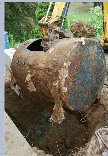
An old underground storage tank being pulled from the ground.
