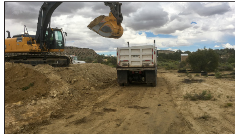
Haul Truck being loaded
