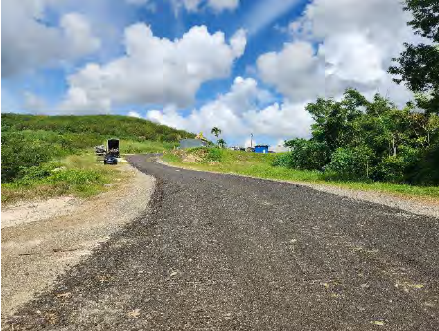
Photograph 13: Partial view of the landfill entrance at the southern portion of the landfill facility, where a berm and inlet grate is recommended to be constructed to redirect runoffs to the south pond.
