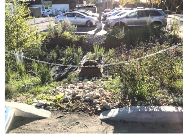
Parking lot infiltration MN Pollution Control Agency
