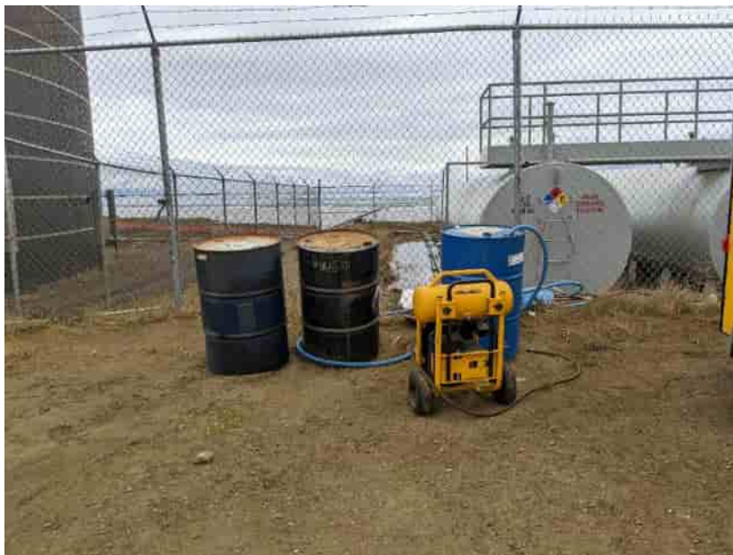
Photo No. 2 – Waste oil/water mixture staged temporarily on the east edge of the Utility Tank Farm outside the fence line. This photograph was taken during cleanup of a fuel spill within the Utility Tanks' secondary containment (HWMU-4). 22 June 2022
