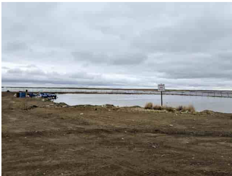
Photo No. 1 – Sewage lagoon in the eastern portion of the fenced-in landfill area, which is not part of a waste management unit. 22 June 2022
