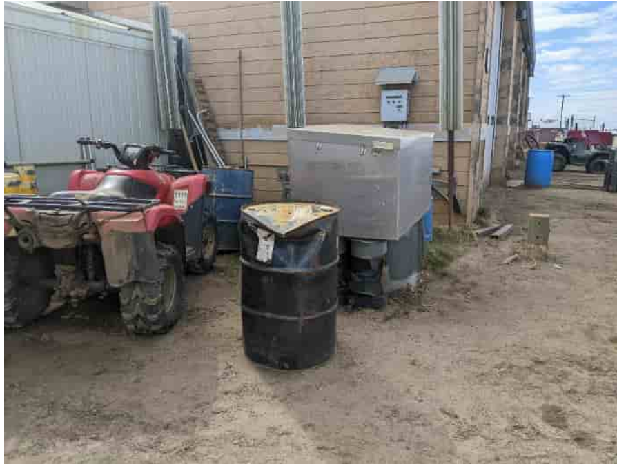
Photo No. 11 – Drums stored south of the hallway connecting the HEMF and O&M buildings (HWMU-3). 21 June 2022
