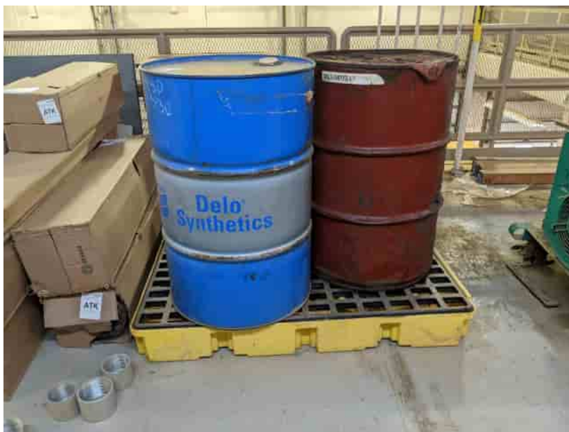
Photo No. 1 – Two drums of waste materials stored on the mezzanine of the USDW building, in containment, above the garage bays (HWMU-1). 22 June 2022
