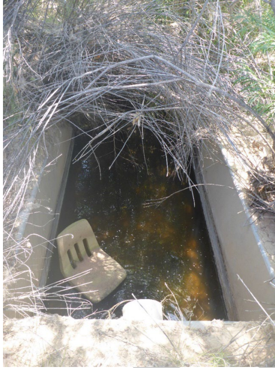
Outfall 001 where final effluent enters a concrete chamber and flows to the Moenkopi Wash (circa June 2023 inspection report)
